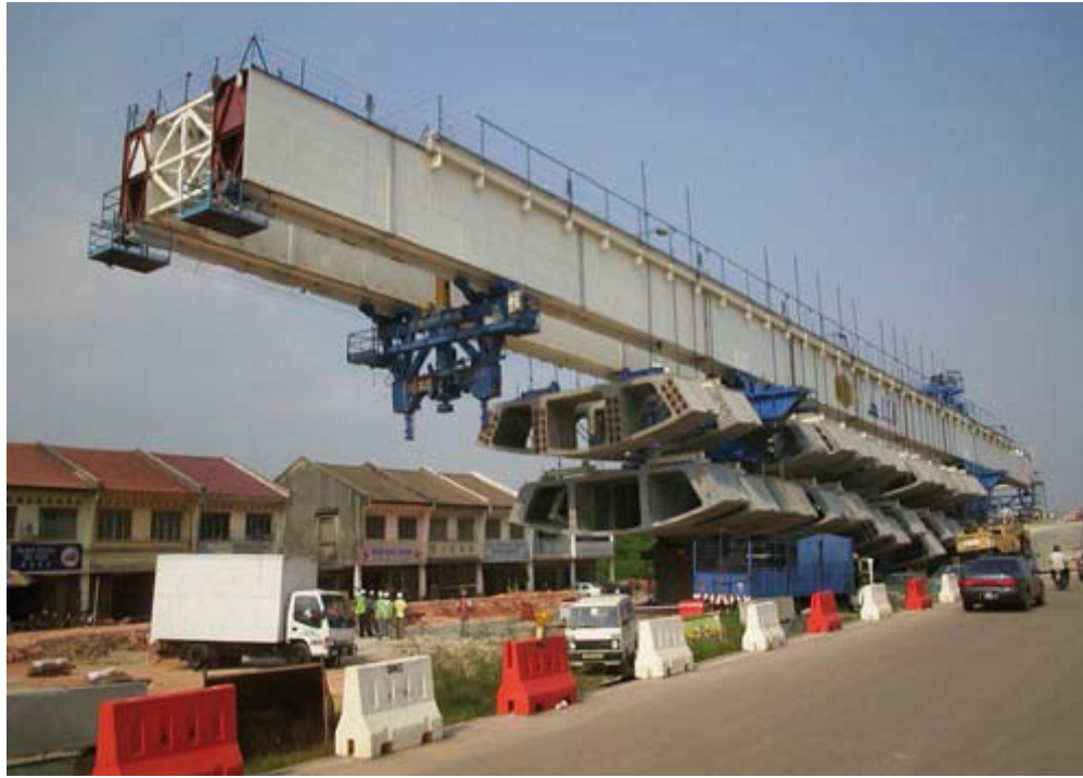
Segment PSC bridge launcher 1500 t in Penang (Malaysia)
