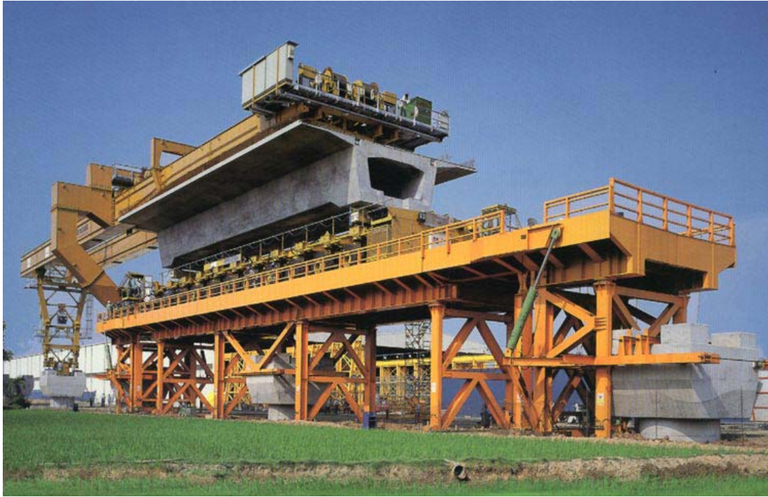
FSM launcher + Tyre carrier 660 t in Taiwan
