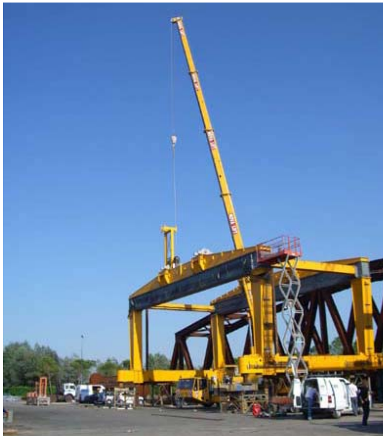
Precast yard transporter 250 t in Vancouver (CAN)
