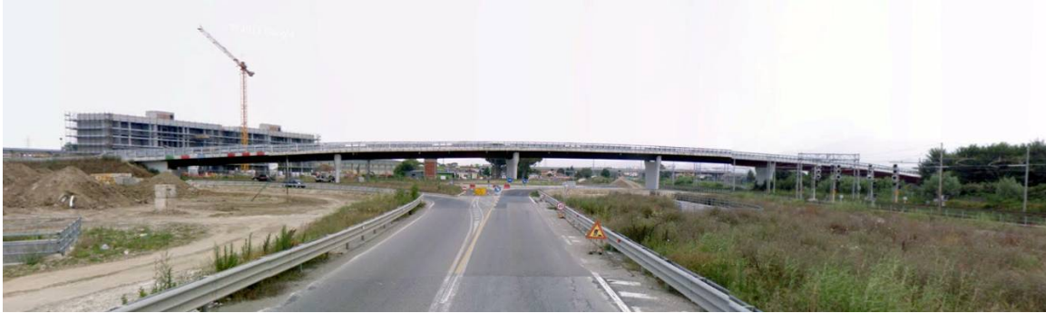
Continuous straight composite steel-concrete bridge.
