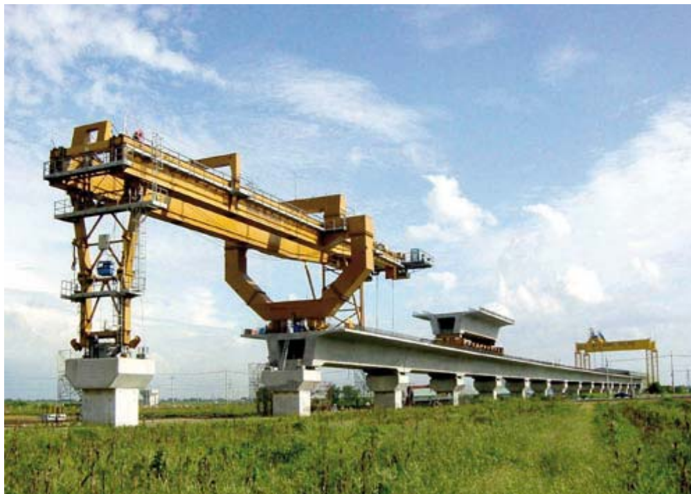
FSM launcher + Tyre carrier 915 t in Taiwan
