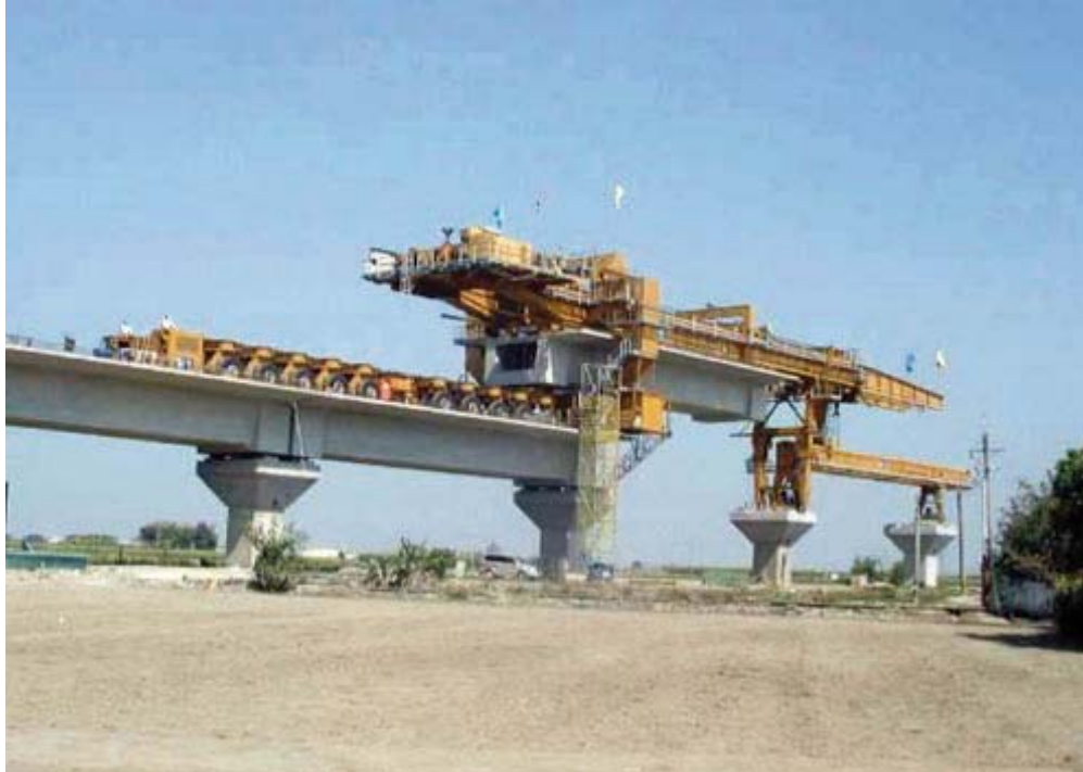
FSM launcher + Tyre carrier 880 t in Taiwan
